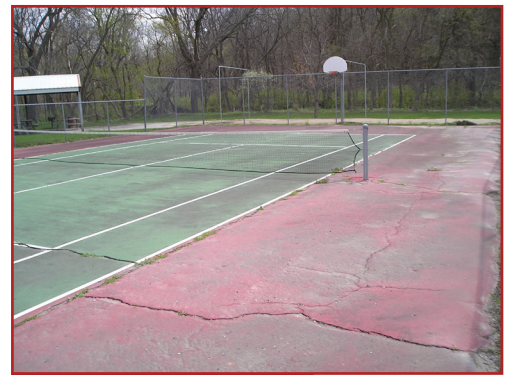
Figure 58: This tennis court may need to be reconstructed because regular maintenance was deferred
