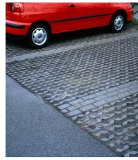
Surface lots can use permeable pavers that allow for stormwater to infiltrate into the ground, decreasing runoff and flooding.
